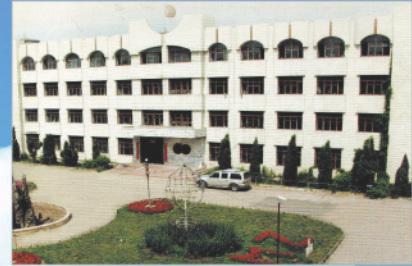
Plant Location : Mudanjiang, China
