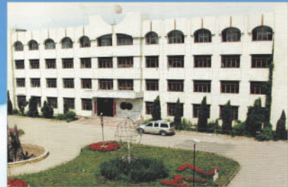
Plant Location : Mudanjiang, China
